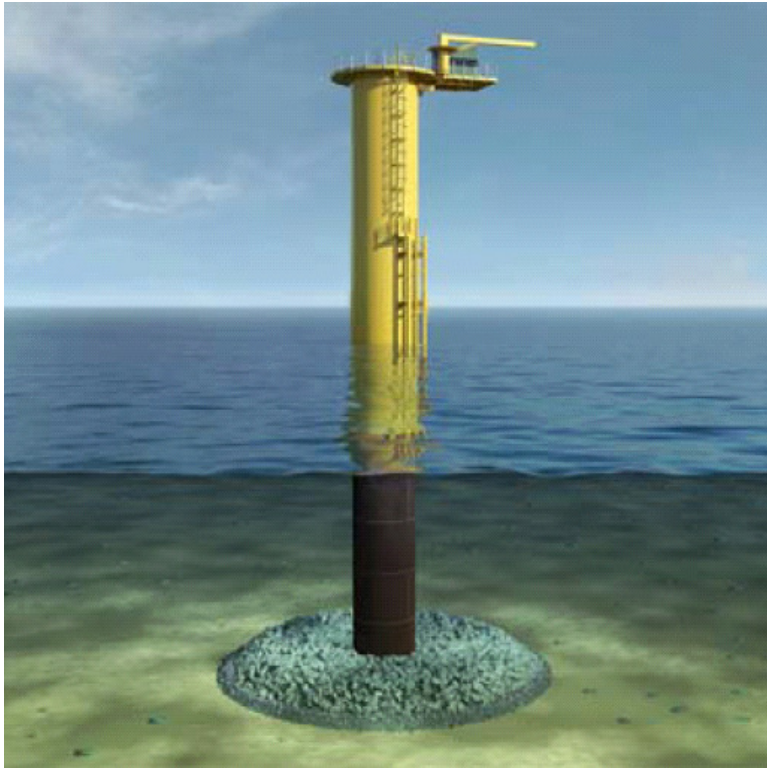
Monopile foundation with transition piece and scour protection. Flange height above sea level approximately 20 meters. 200-300 tons
