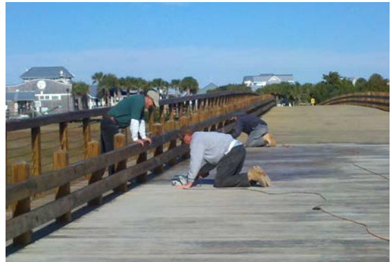
Village of BHI's Public Works staff work to prepare the transmarsh timber bridge's surface for a protective sealant. The bridge was closed from late October through Thanksgiving for staff to complete the work.
