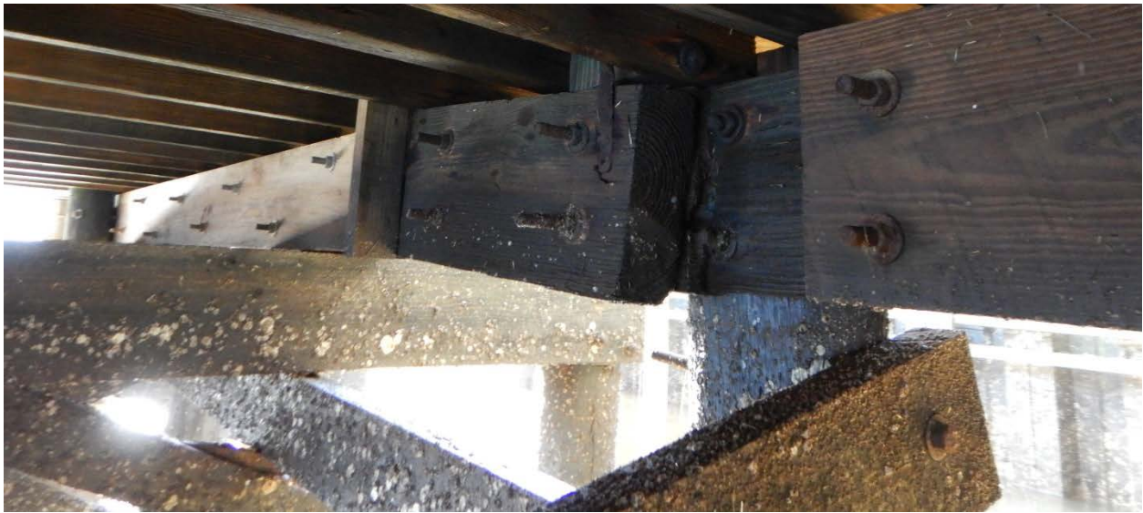
FIGURE 2-26: UNDERDECK VIEW OF TIMBER STRINGER
