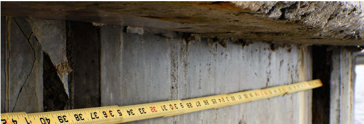
FIGURE 2-17: DISPLACED CONCRETE SHEET PILES AT BULKHEAD REPAIR SECTION
