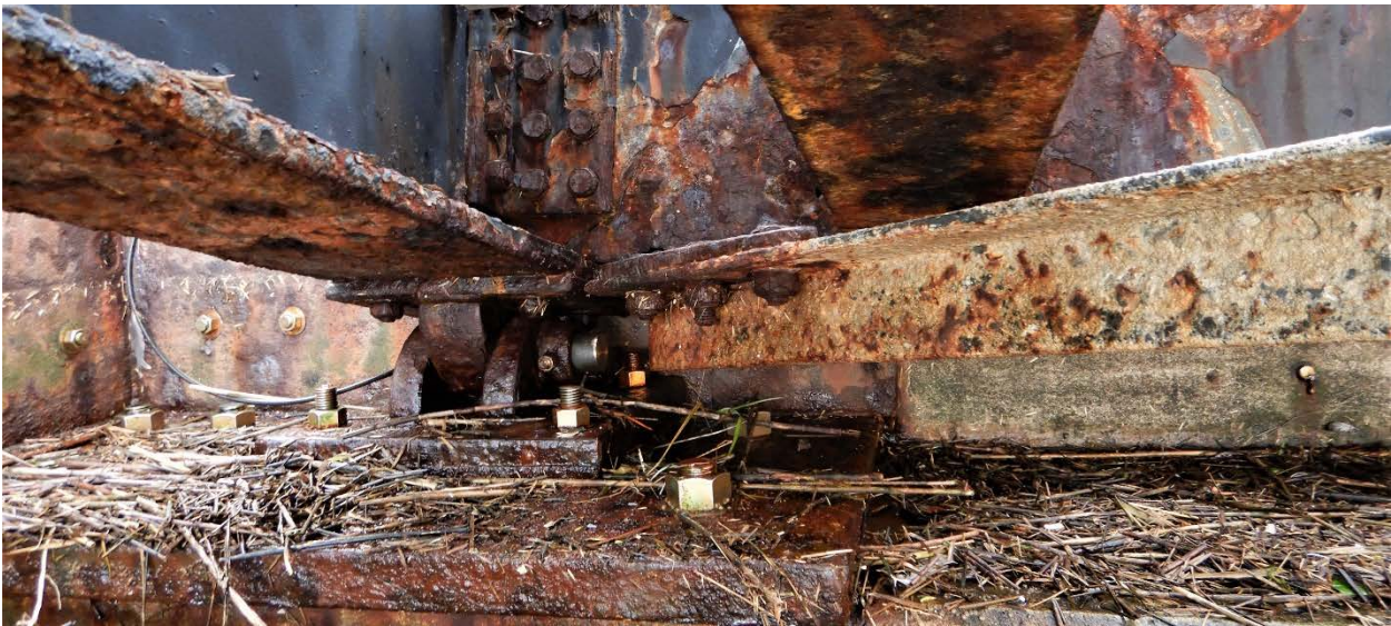
FIGURE 2-21: BHI BARGE RAMP STEEL FRAMING MODERATE CORROSION
