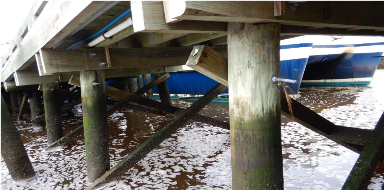
FIGURE 2-6: DPM MAINTENANCE FIXED PIER TIMBER PILE BENTS
