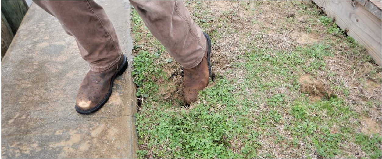
FIGURE 2-15: TYPICAL SINKHOLES BEHIND WALL
