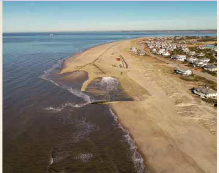
Sand dredging on South Beach. Photo courtesy Village of BHI.
