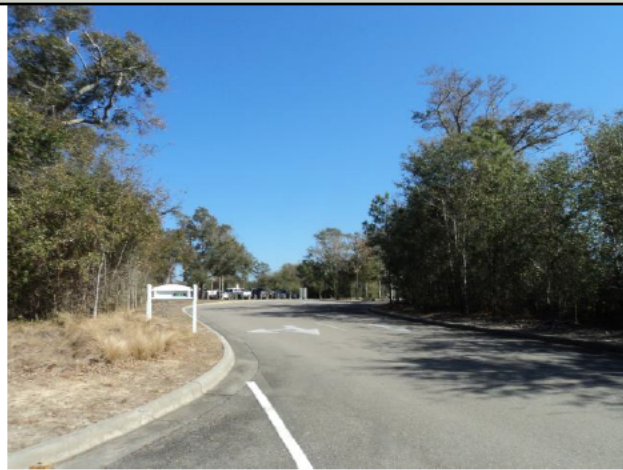
Typical Access Road
