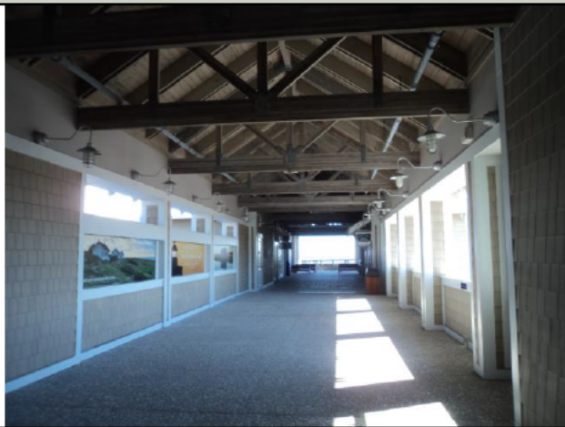
Covered Passenger Deck
