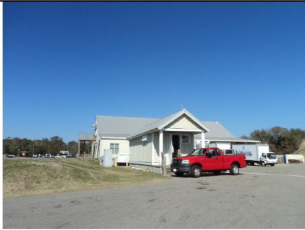
Computer Server Building
