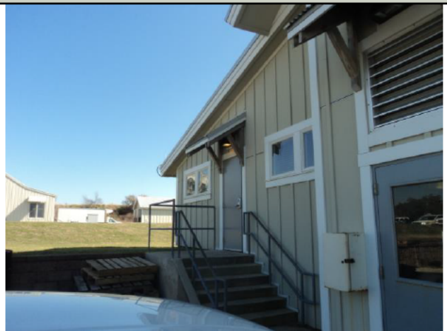
Ferry Repair Building
