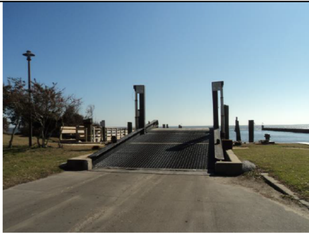
Barge Loading Area
