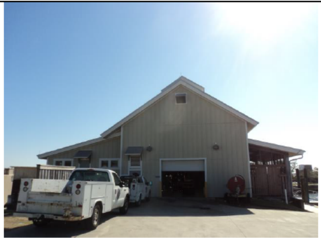
Ferry Repair Building
