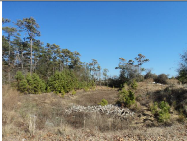
Storm Water Retention Pond
