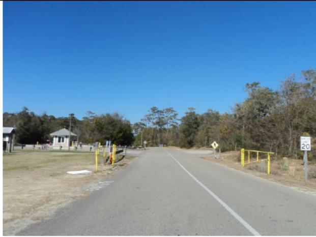
Typical Access Road
