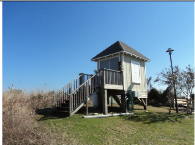
Barge Lift Mechanical Building
