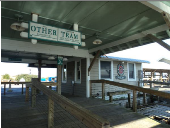
Covered Passenger Deck
