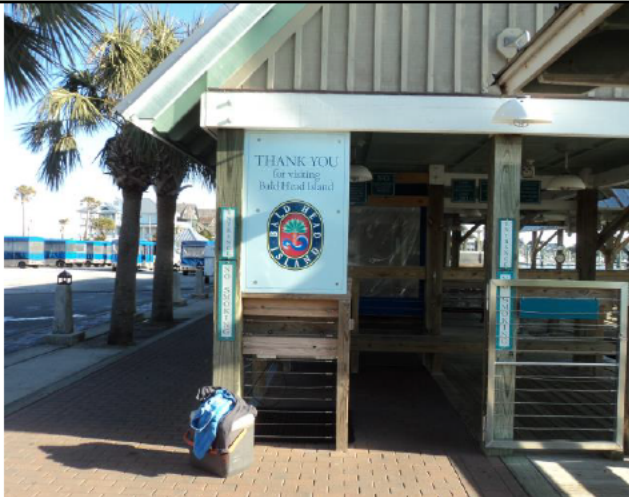
Side View Main Building
