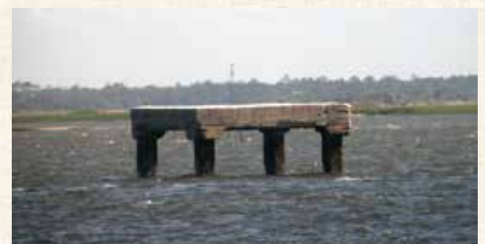
Concrete support for quarantine station watertower. Courtesy of http://federal-point-history.org
